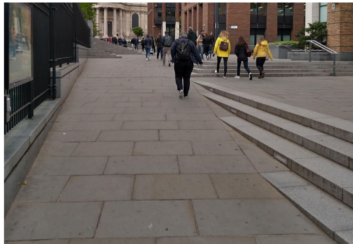
Accessible steps - a gentle slope with elegantly intersecting steps, leading up to St. Paul's Cathedral, depicting the benefits of accessibility by design.
